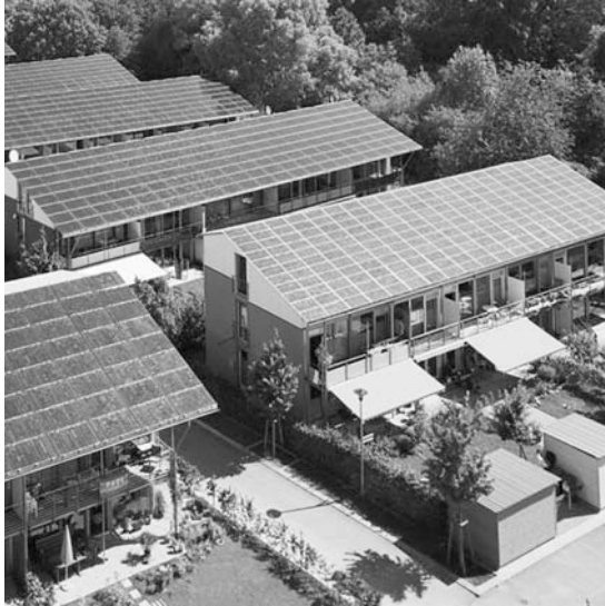
FIGURE 1. The solar estate, “ Solarsiedlung Freiburg am Schlierberg. ” 59 plus-energy terrace houses, nine of them on the flat roof of an office block. Source: Büro Disch.
